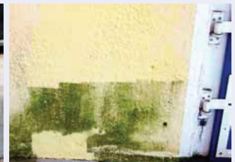
moss-covered coat of paint
